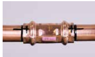
3. Mark the completed joint
