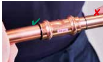
8. Insert the tube fully into the fitting. Ensure tube is fully inserted prior to pressing
