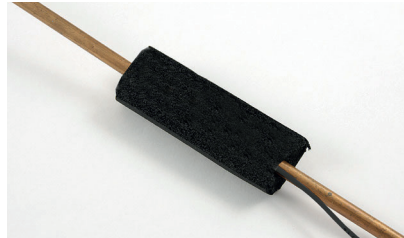
5) Cover the sensor with thermal insulation for at least 10 cm around the end of the cap and the wound cable;
